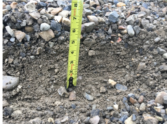
Segregation of material
