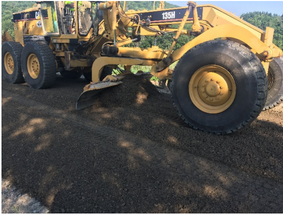
Grader spreading
