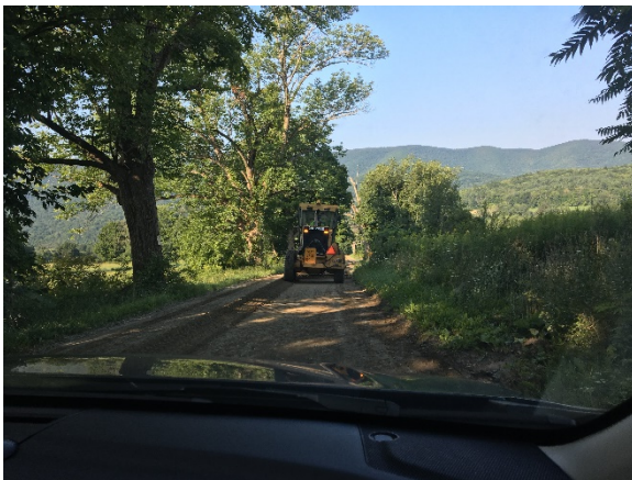
Grader shaping of existing roadway materials
