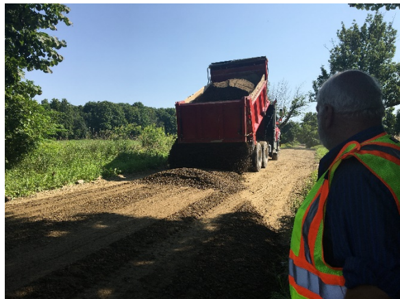
Truck dumped and spread material
