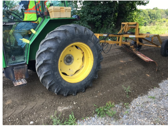
Tractor rake of surface
