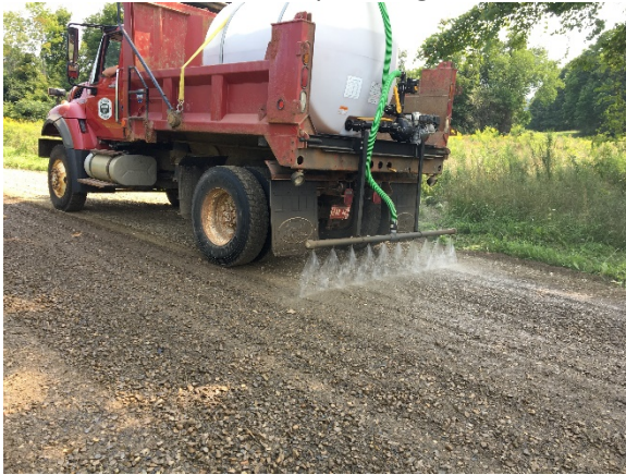
Chloride application
